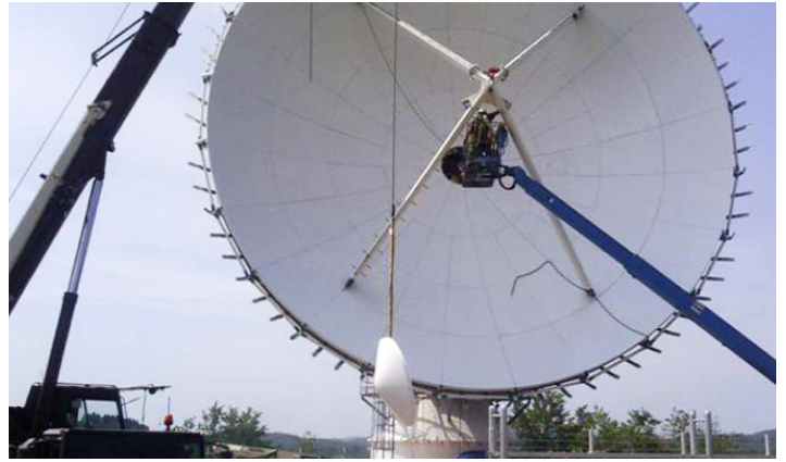
GOES-R RBU Antenna Construction
