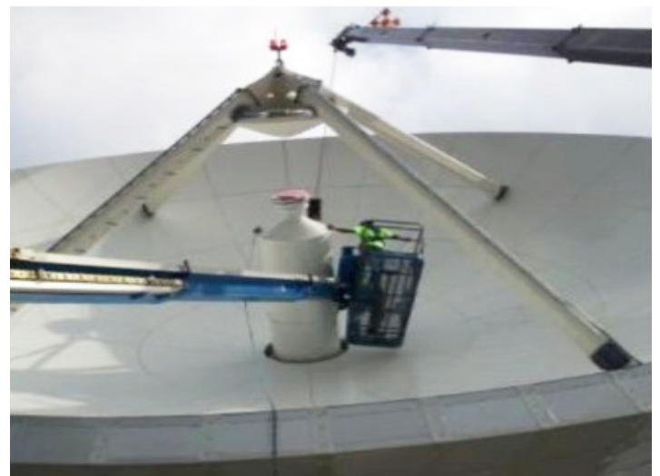
RBU R-2 antenna feed installation. Credit: Harris Corporation
