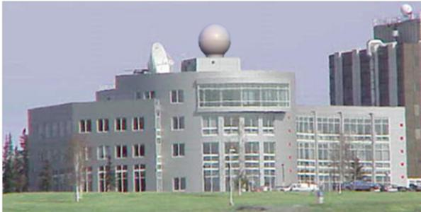
**Figure 1.** UAF-GINA's X-band receiving station antenna is inside the radome in the center of the photograph. The large, fixed dish to its left is the NWS Fairbanks WFO's NOAAport antenna. The small radome in the upper right holds an L-band antenna.
